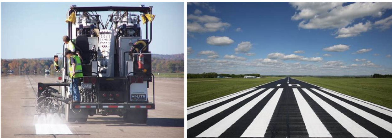
Figure 8. Industrial use of glass beads in reflective paint for airfield markings (AviationPros, 2012; Hi-Lite Airfield Services, 2019).
