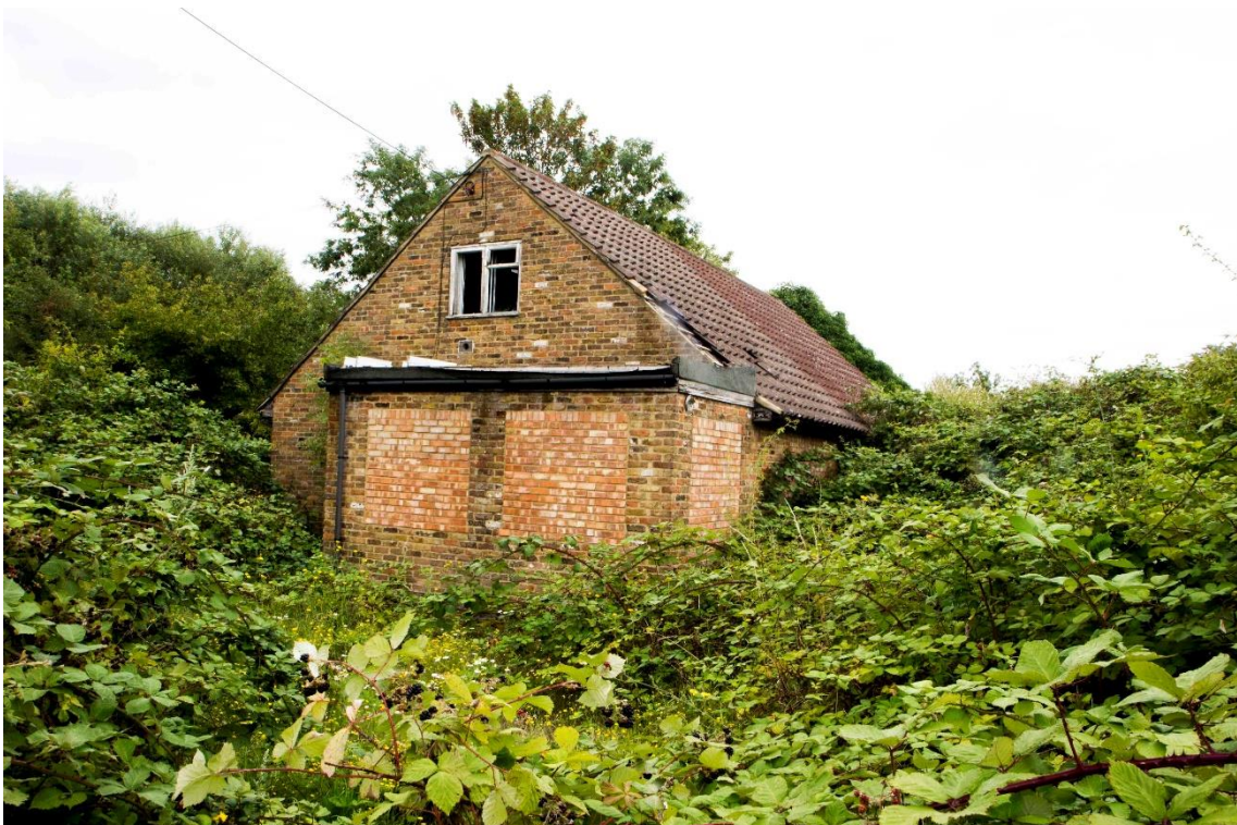
Figure 18. Nicholas Ferguson. Bricked up building, Stanwell Moor.
