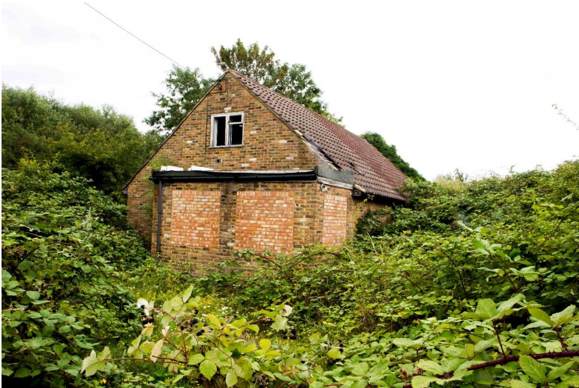
Figure 17. Nicholas Ferguson. Bricked up building, Stanwell Moor.
